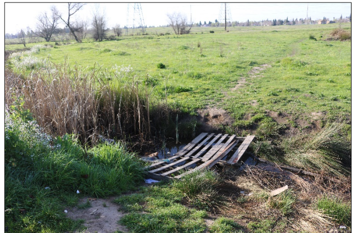
Example of user-created bridge over Kaseberg Creek East Branch constructed of pallets.
