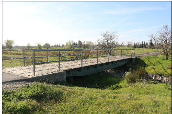
Existing bridge over seasonal creek in the Silverado Oaks Open Space just south of the Study Area.
